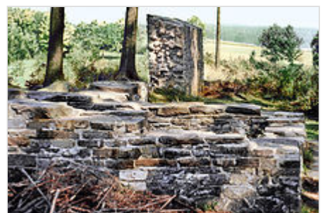
At WP 12/77, part of the limes wall has been fully reconstructed ( Mahdholz )
