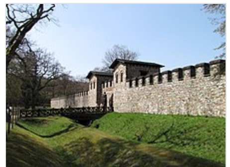
The Saalburg . Built 1899–1907, the site is the most significant attempt to reconstruct the archeological past. The southwest corner built by Louis Jacobi in 1885 with merlons at the wider and thus correct intervals, had to be replaced during the full reconstruction, probably at the behest of Emperor William II, with merlons spaced at the medieval interval, which is thus wrong. [1]
